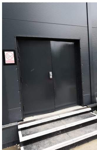
fire exit doors exterior
