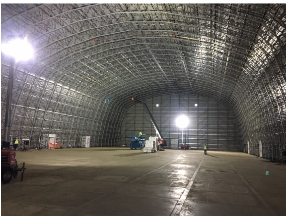
ITV Interior Production Load In
